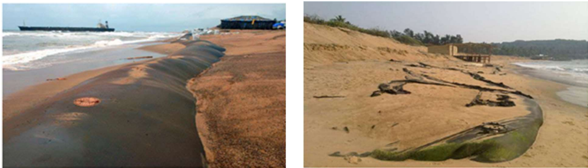
Figure 16-failure of Geotubes at Candolim beach in India (R Parab et al. , 2019).
