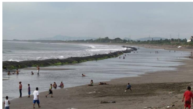
Figure 1: Geotubes on the beach in Corinto (Source: Städtepartnerschaftsverein Köln/Corinto)
